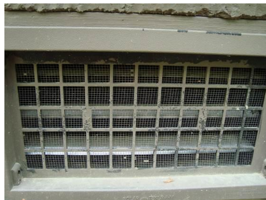
The mesh on this foundation vent will help prevent embers from entering under the house.
